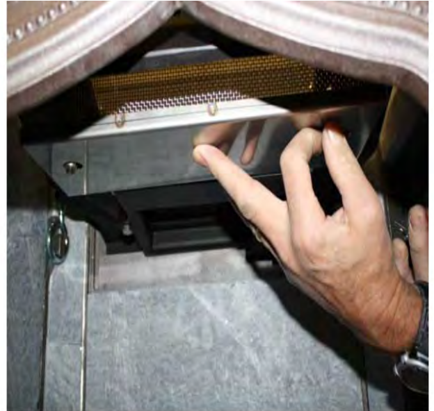
Scoop plate is sandwiched between the top roll pin and the cotter pin.
