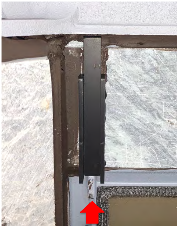
3. Align the two spacers with the cast iron that juts out on the right & left of the window.
