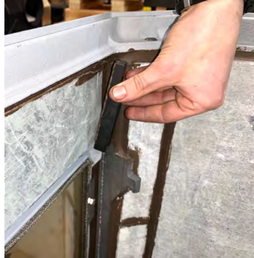
2. Attach the spacers to the stone above the glass.
