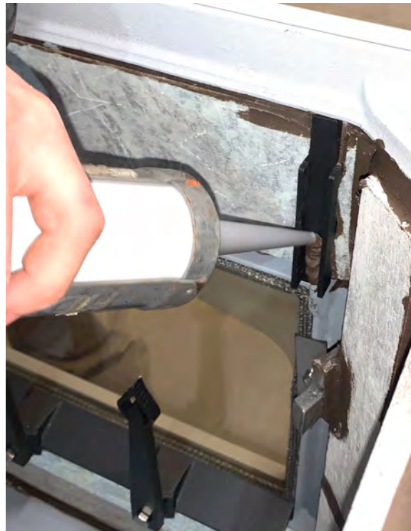
4. Fill the channel on each spacer with furnace cement.
